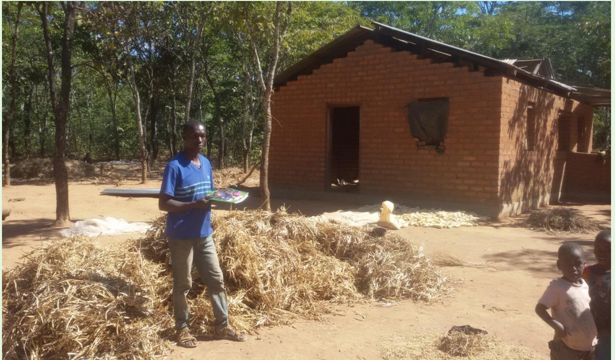
Mr. Sylvester Mukuka with 2 of his children, stands amid husks of shelled beans (2016 harvest) and his new house which is under construction. Photo: Self Help Africa
