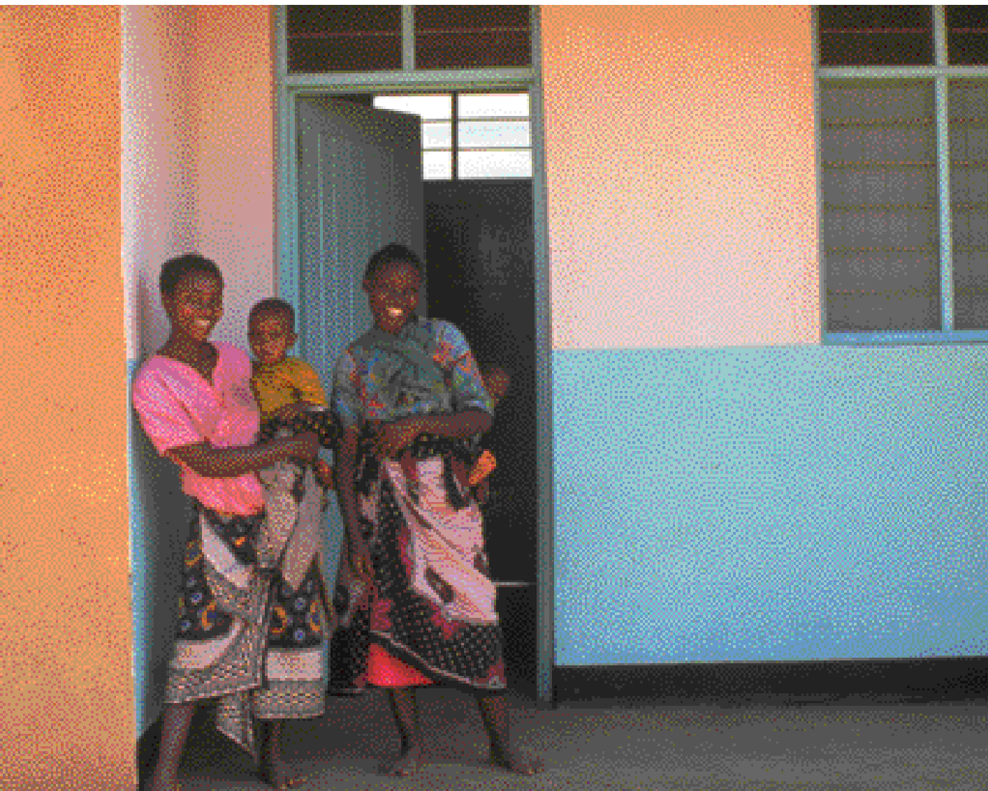
Housing for teachers at Italagawe primary school, Kilosa district, Tanzania © Carol Lee
