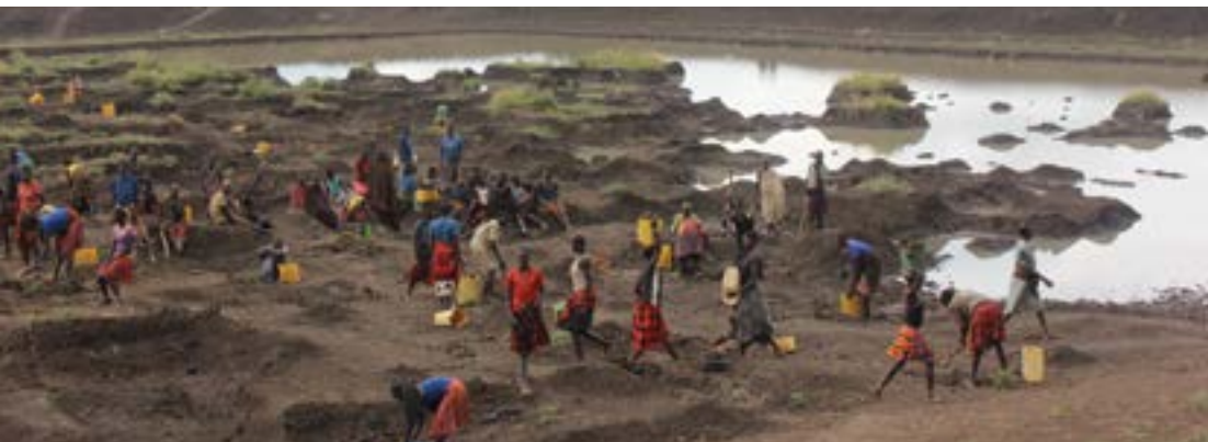
Community members digging a valley dam, Kotido District, Karamoja. Photo: Irish Aid
