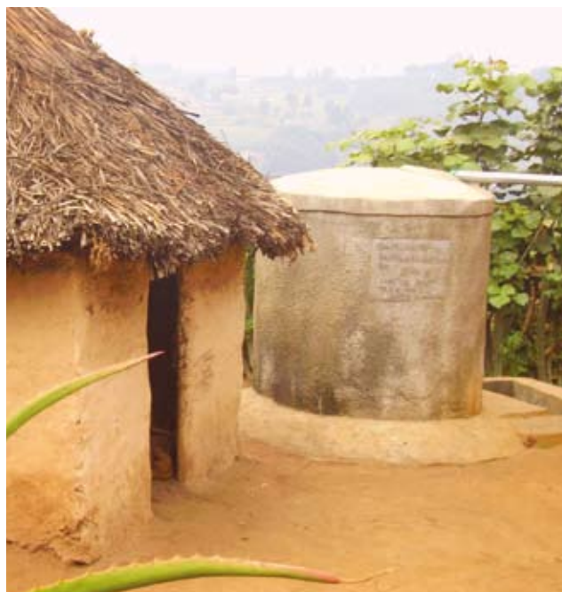
A water tank in Kagarama, Uganda, constructed by the community under the Diocese of Kigezi's Water and Sanitation programme supported by Tearfund and financed by Irish Aid
