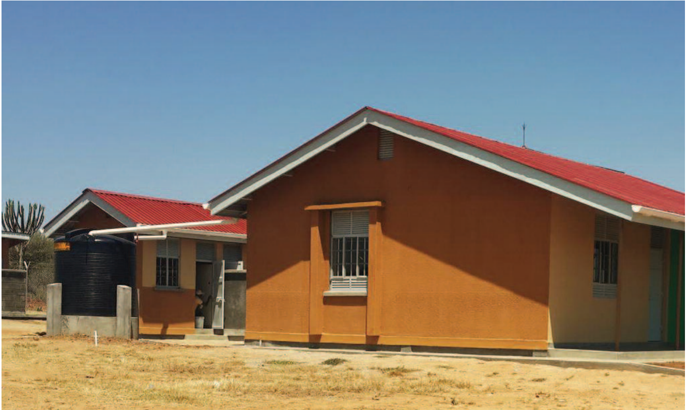
Katikit Primary School, Amudat District, Karamoja which was constructed with Irish Aid funding under the Karamoja Primary Education Project. Photo: Irish Aid
