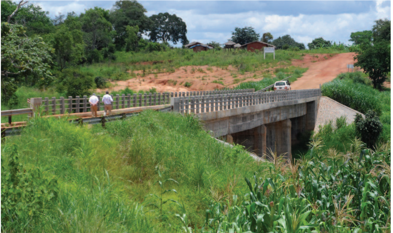
Luchimua Bridge in Niassa province, built with Irish Aid funds to improve land communication between Majune and Mandimba districts. Photo: Irish Aid
